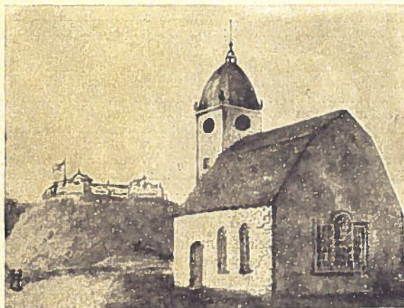
ST. PETER'S CHURCH, 1715 (Fort Frederick in the Background)
